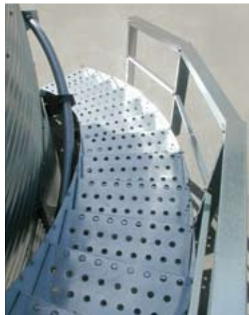
Stairway can be used with stiffened or unstiffened bins, or bins with wind rings.
