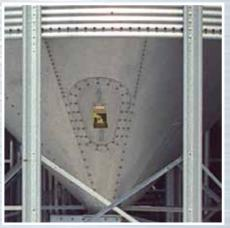
Brock's ACCESS PLUS<sup>®</sup> Hopper Access Door gives easy access to the interior of the holding bin.
