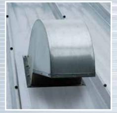
Gravity roof ventilators provide free air movement into the bin. Elbow-style (shown) and round mushroom-style vents are available.
