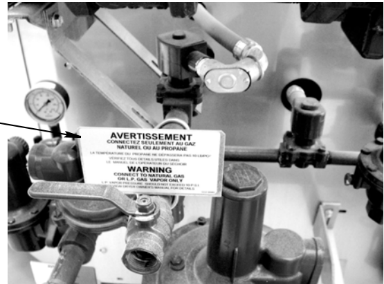
Figure 1, above. Fuel WARNING Plate LP Gas Vapor 5537-00049
