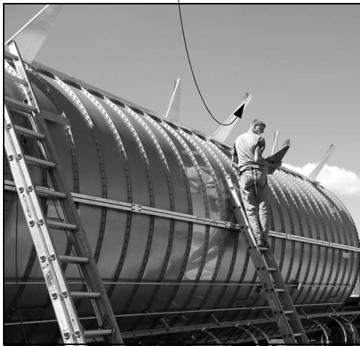
Figure 9. Install Walkway Arms
