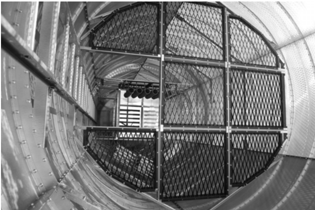
Figure 69. Inside Ladder Through the Service Platform Opening
