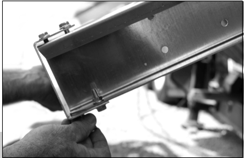
Figure 14. Walkway Posts: DO NOT TIGHTEN at this time!
