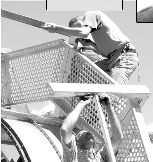
Figure 14. Walkway Posts: DO NOT TIGHTEN at this time!
