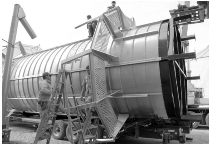
Figure 6. Right: Walkway Installation on Horizontal Tower
