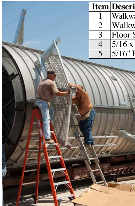
Figure 13. Connect Adjacent Floor Sections
