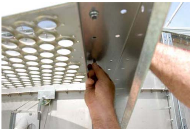
Figure 12. Walkway Floor Sections
