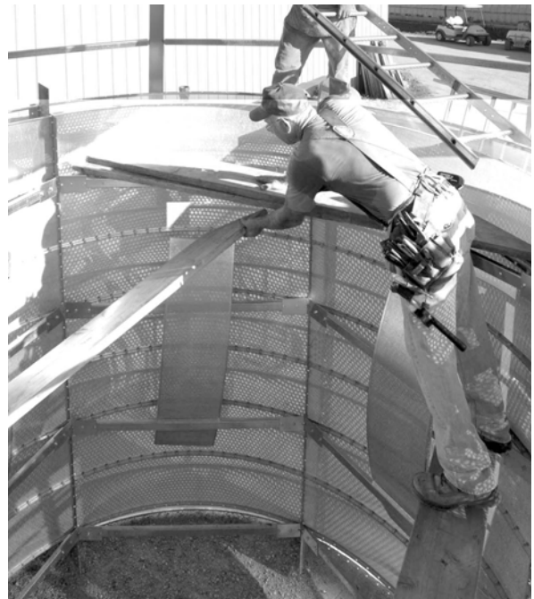
Figure 72. Top Inside Ladder Installation in the Tower
