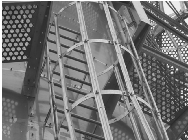
Figure 70. Inside Ladder with Cage
