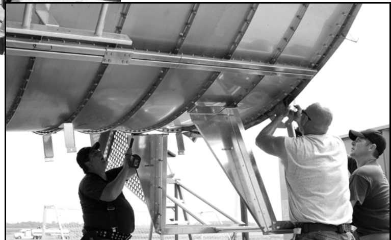
Figure 21. Install Walkways at Tower Trailer FIRST STAGE Lift
