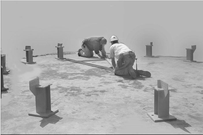
Figure 29, above. Stub Leg Fixture Placement (12 on 18' BCT)
