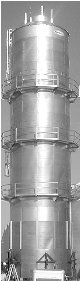
19 Rings with Upper Stiffeners
