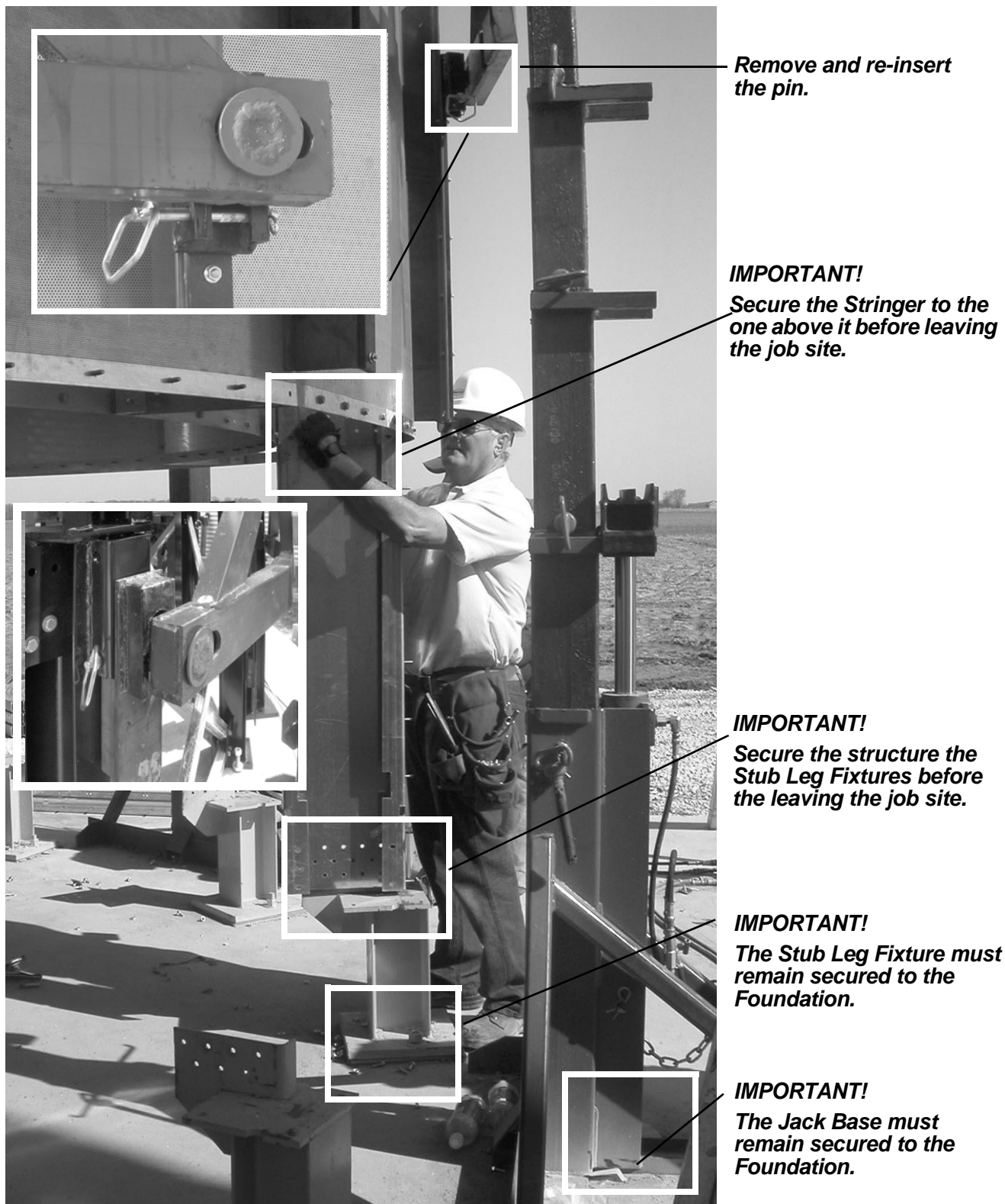
Figure 33. Hydraulic Jack Usage
