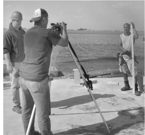
Figure 22. Shim (above) the Pad to Level
