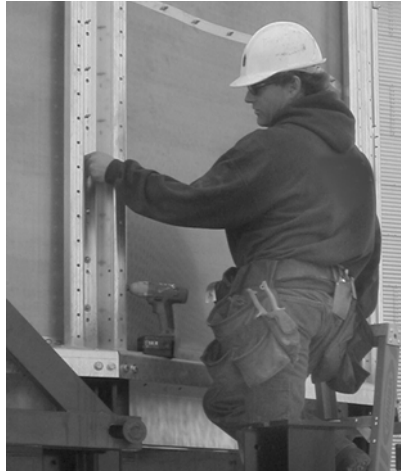
Figure 112. Replace Stiffener Hardware
