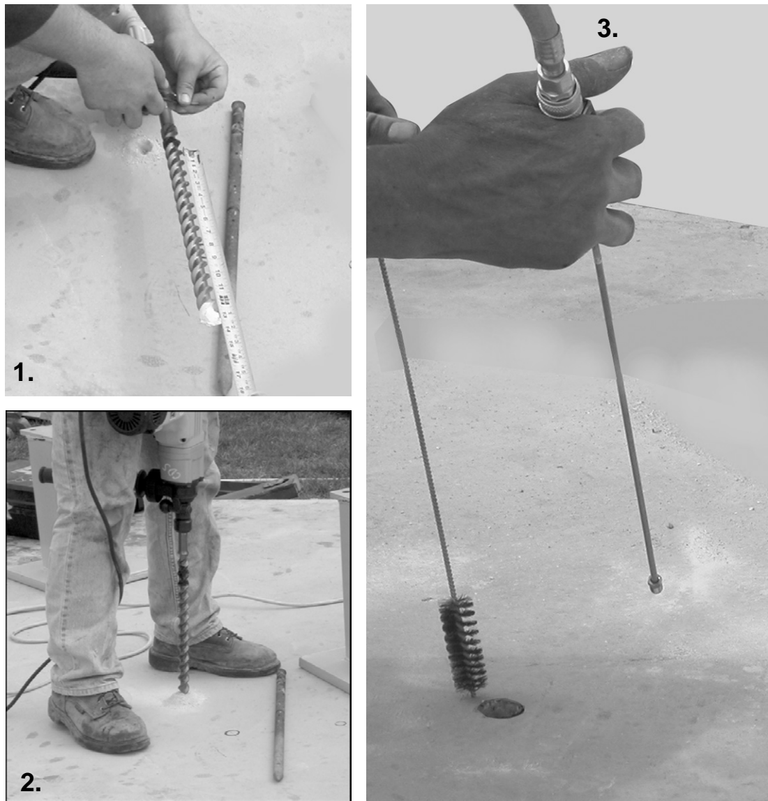
Figure 26. Drill Anchor Bolt Holes
