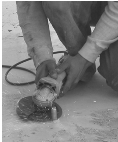
Figure 121. Patch Bolt Holes
