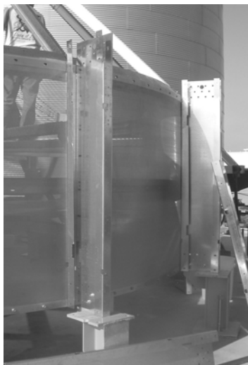
Figure 57. Starter Ring Inside (18' shown)
