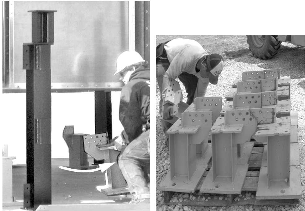
Figure 94. Remove Stub Leg Fixtures
