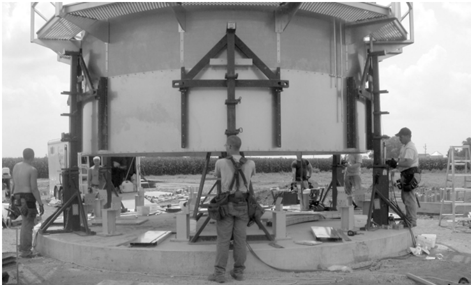
Figure 38. Raising the Tower with Hydraulic Jacks
