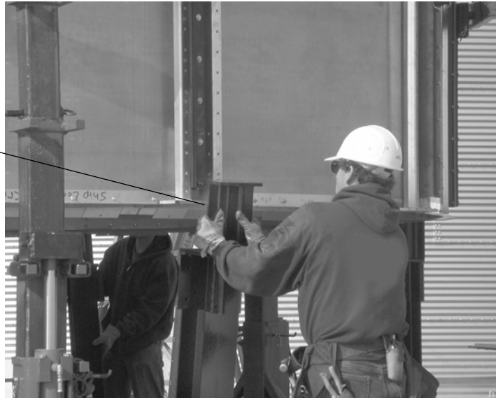
Figure 96. Install Upper Leg Weldments
