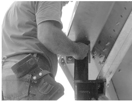
Figure 103. Beam Bracket Placement (Item Table on facing page.)
