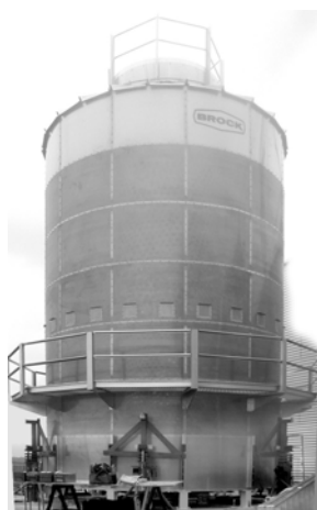
7 Rings, (Jacks lowered to build Walkway)
