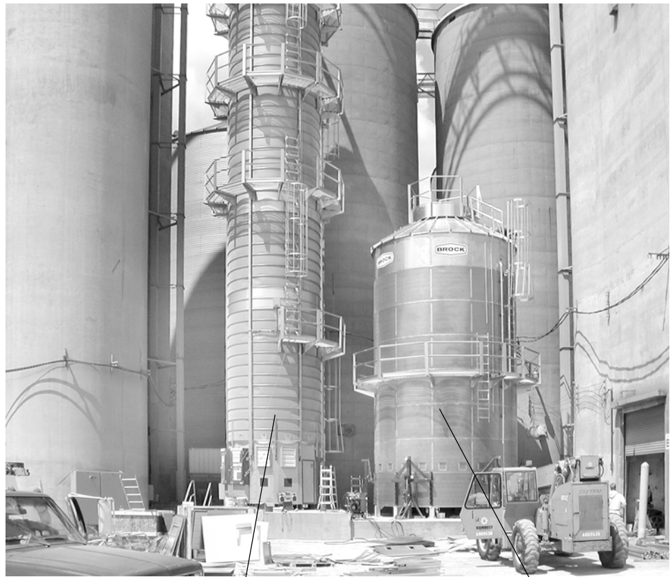
Figure 7. Left: BROCK® MEYER® Tower Dryer Right: BROCK® BCT Dryer 18' (construction)
