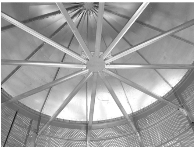
Figure 71. Tower Roundness Fixture Remains
