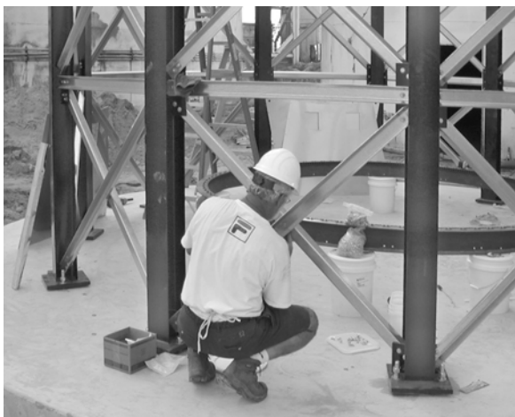
Figure 116. Lower X-Braces
