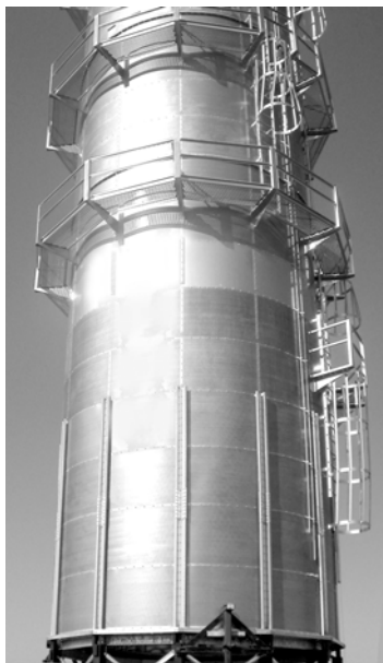
Figure 86. Bottom Stiffeners
